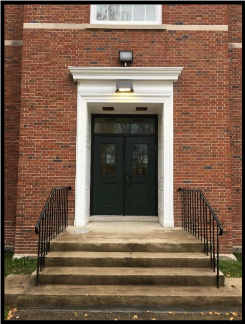
New Exterior Doors
